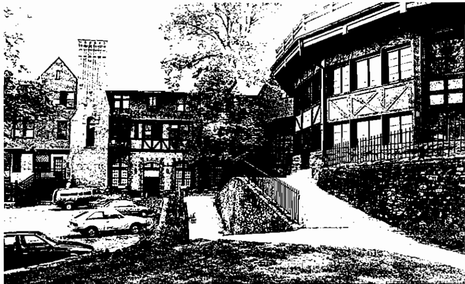
Manor Inn, Asheville. During the demolition delay period imposed by the Asheville-Buncombe County Historic Resources Commission, local preservationists purchased and stabilized the landmark Manor Inn. They ultimately attracted a developer, who has restored the buildings as a successful apartment complex.
