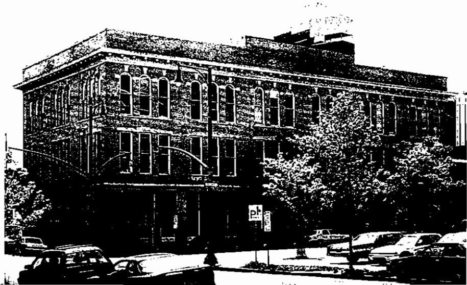
Montague Building, Raleigh. When the Raleigh City Council condemned the 1912 Montague Building for code violations in 1976, a group of preservationists volunteered to correct them, in order to preserve this building, which for most of its history housed African American businesses. Local landmark designation in 1979 helped to trigger the listing of the Moore Square Historic District in the National Register of Historic Places. The local designation and National Register listing in turn attracted a developer who rehabilitated the Montague Building for commercial and office use.
