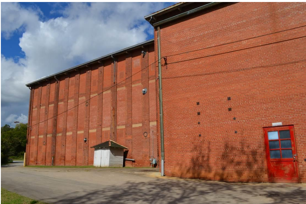
1912 Cannon mill addition
