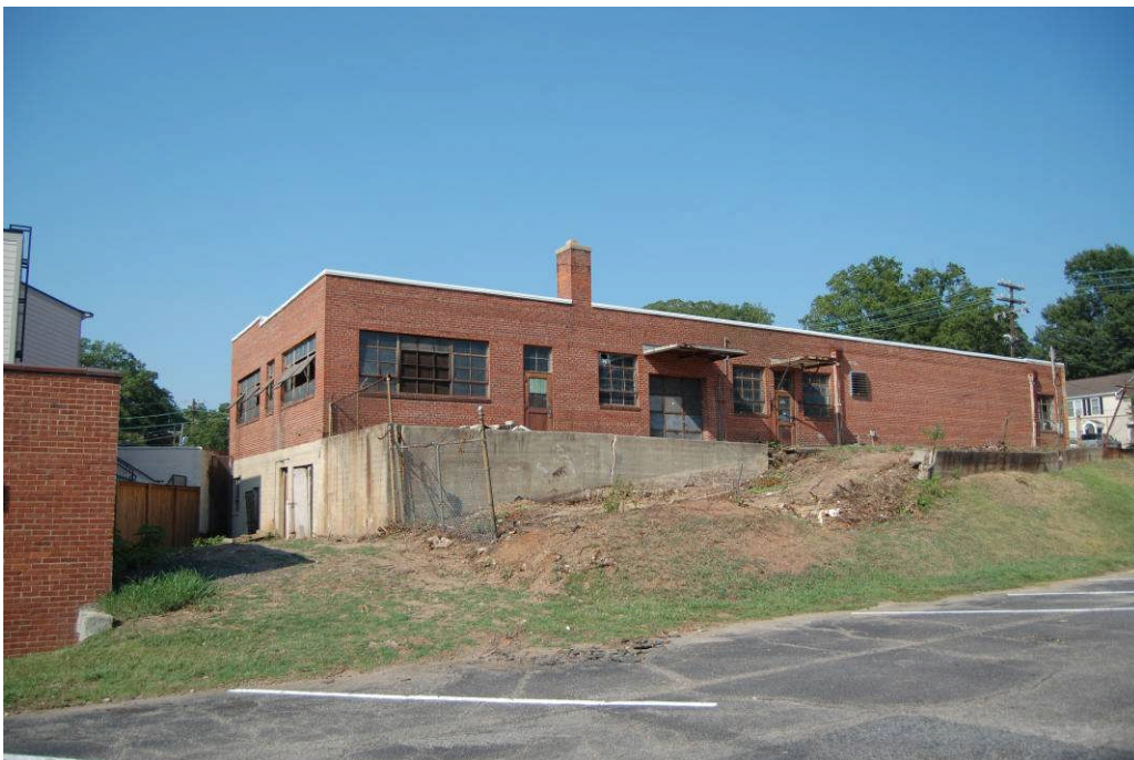
Side and rear view
