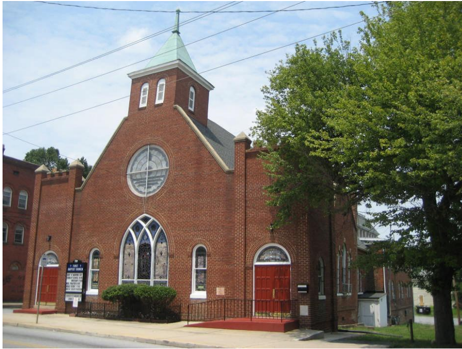
Overall front view
