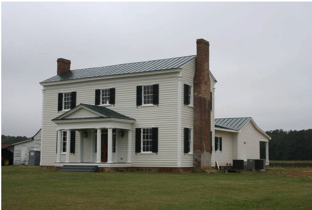
Façade and side view
