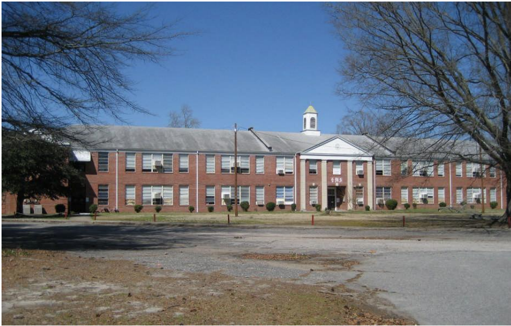
Overall front view
