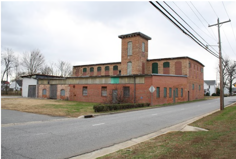
Overall view of mill looking southwest
