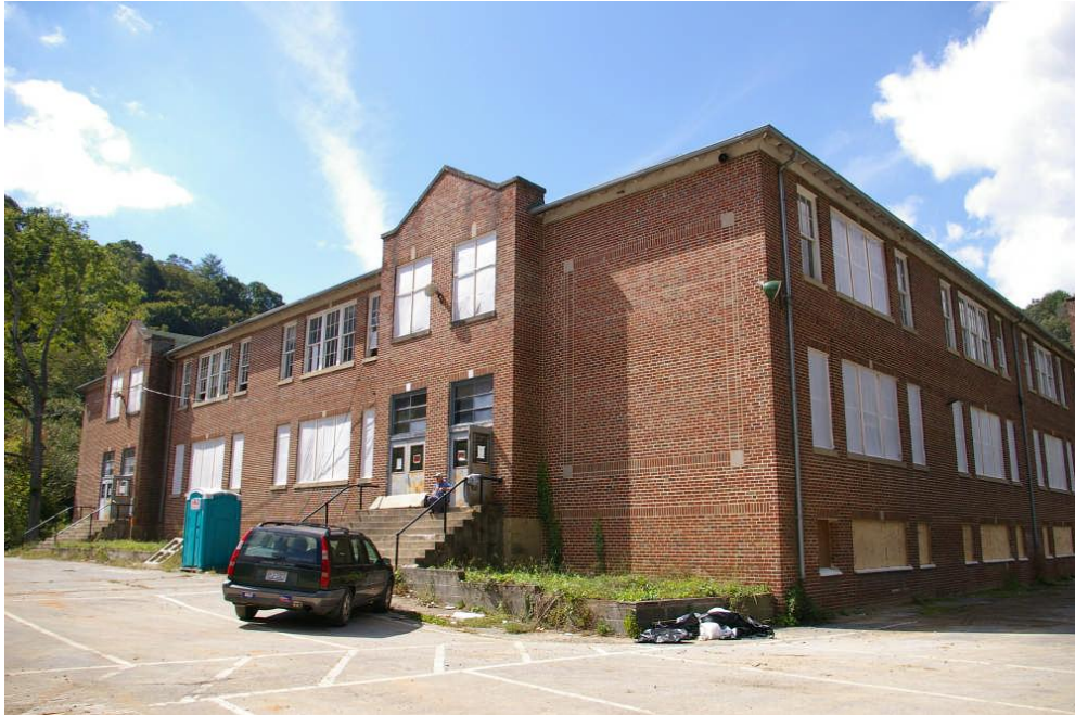
Overall front view
