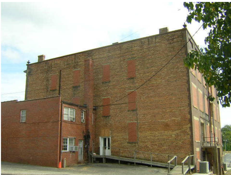
Side and rear view
