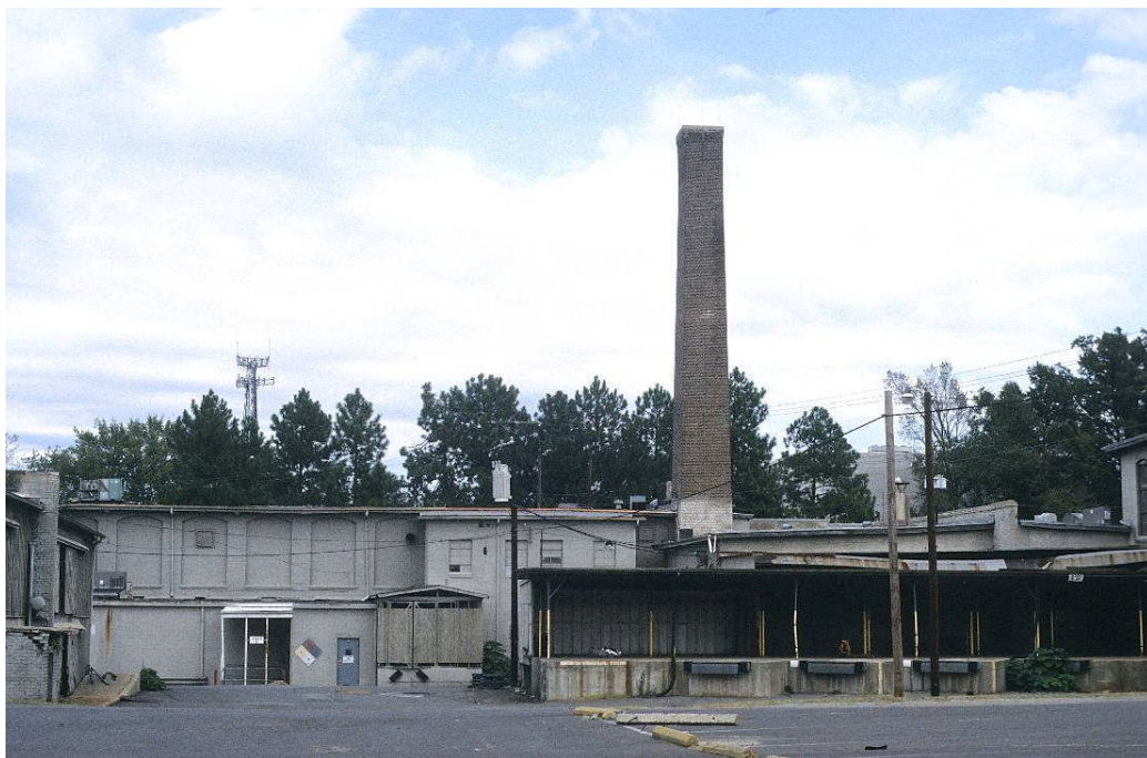
Southeast elevation, ca. 1911 building
