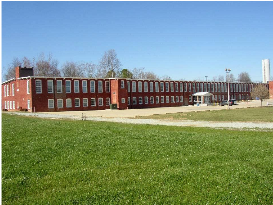
Façade view – southern end
