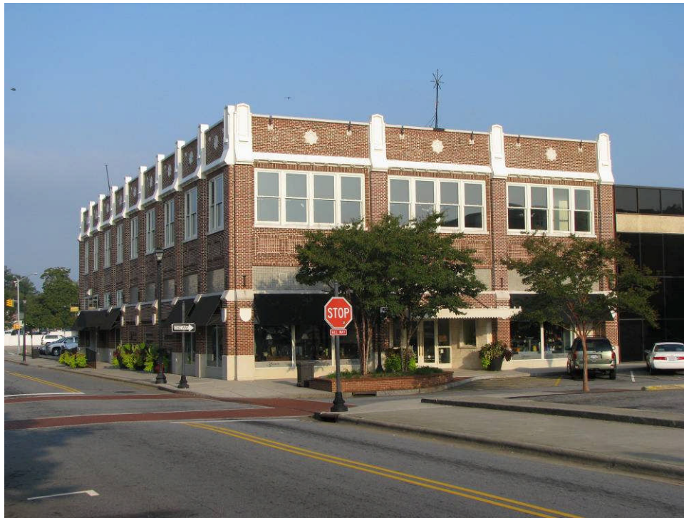
Blount-Harvey Department Store, façade view
