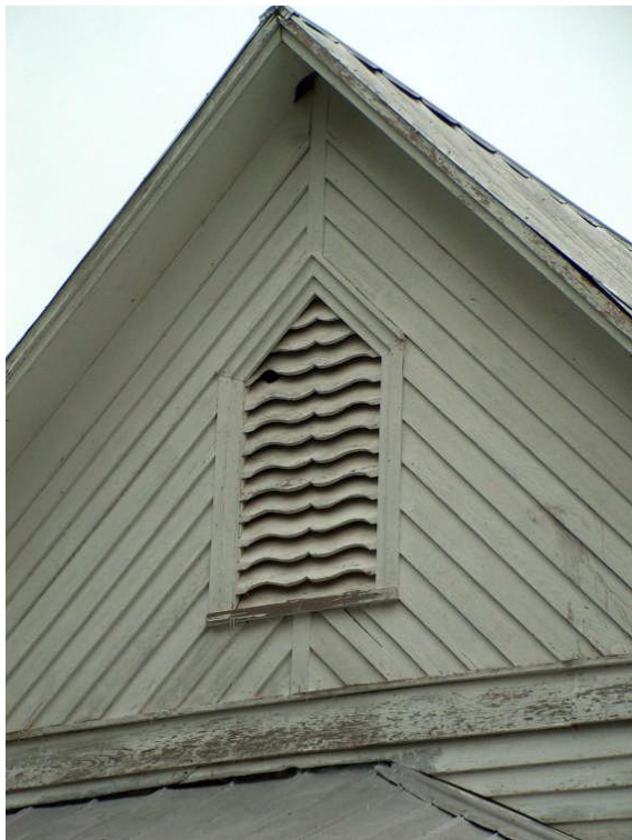
Gable decorative work – detail view
