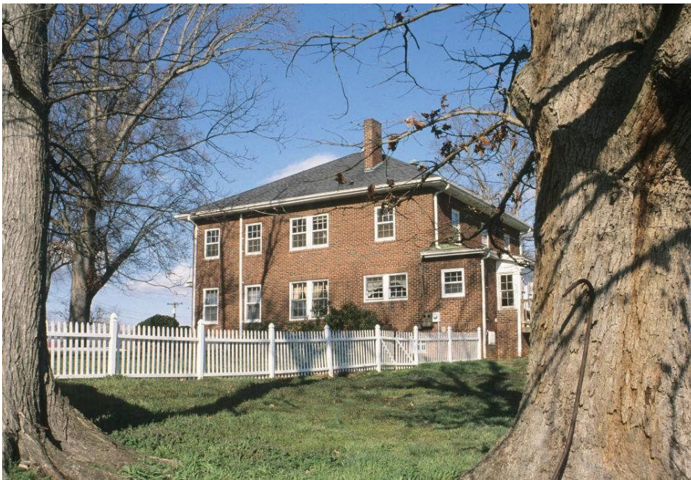
Side and rear view
