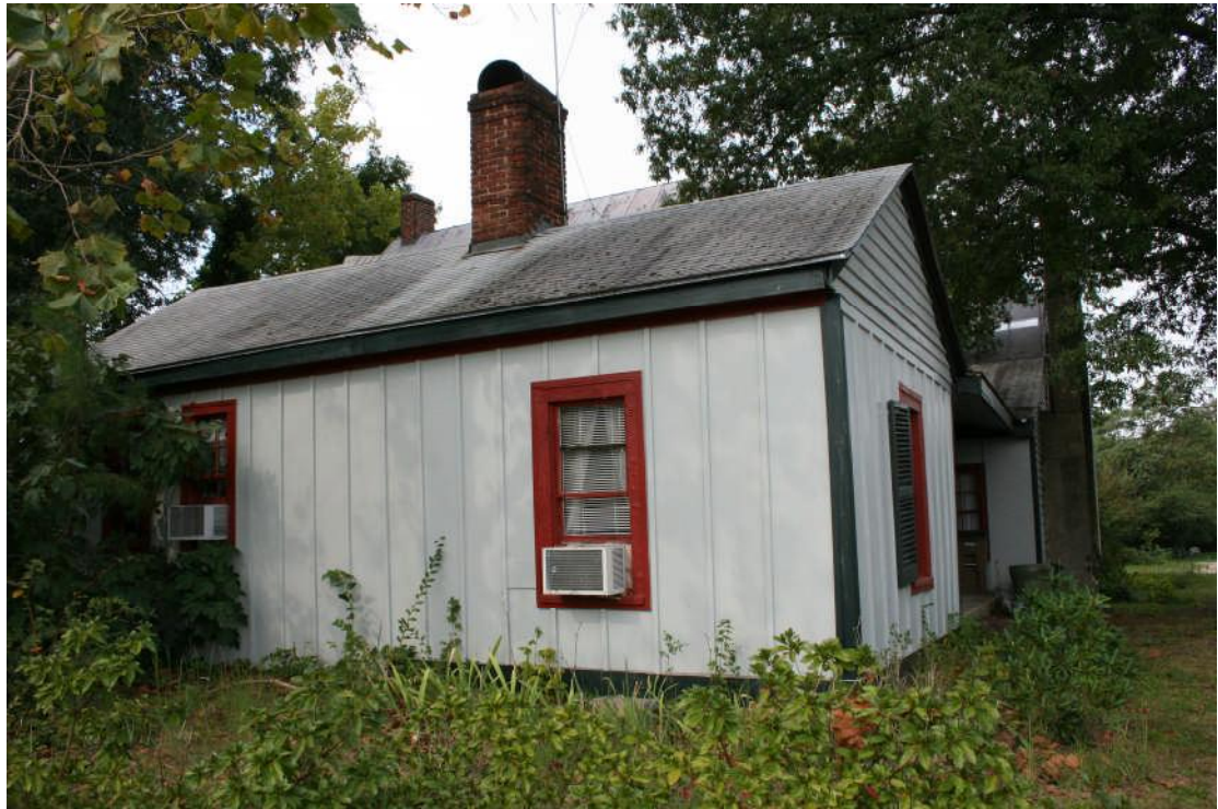
Kitchen/dining building, rear view
