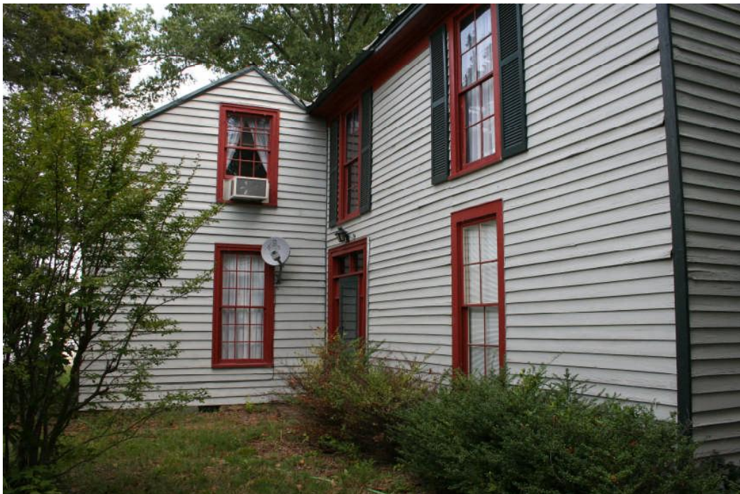
Façade of the ca. 1895 wing on right
