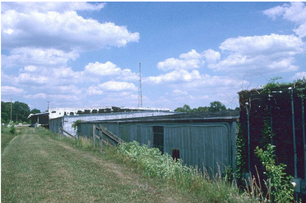
Rear view from railroad right-of-way
