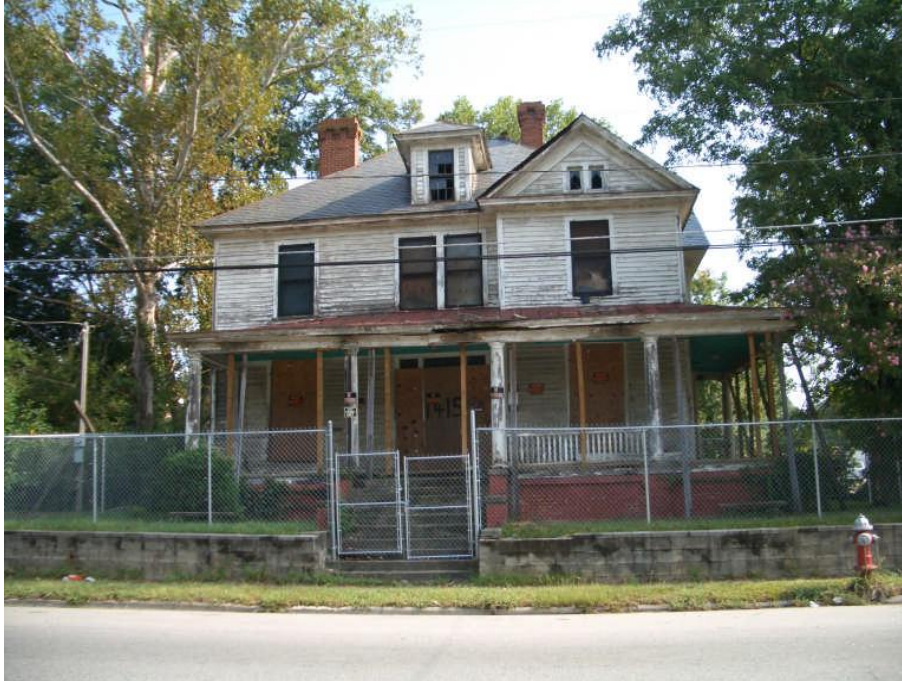
Overall front view
